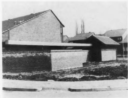
Fig 7 A communal heat pump. The small building on the right houses an air-to-water heat pump, design output 70 kW, to heat a row of 12 houses. The horizontal duct carries the water flow and return mains.
